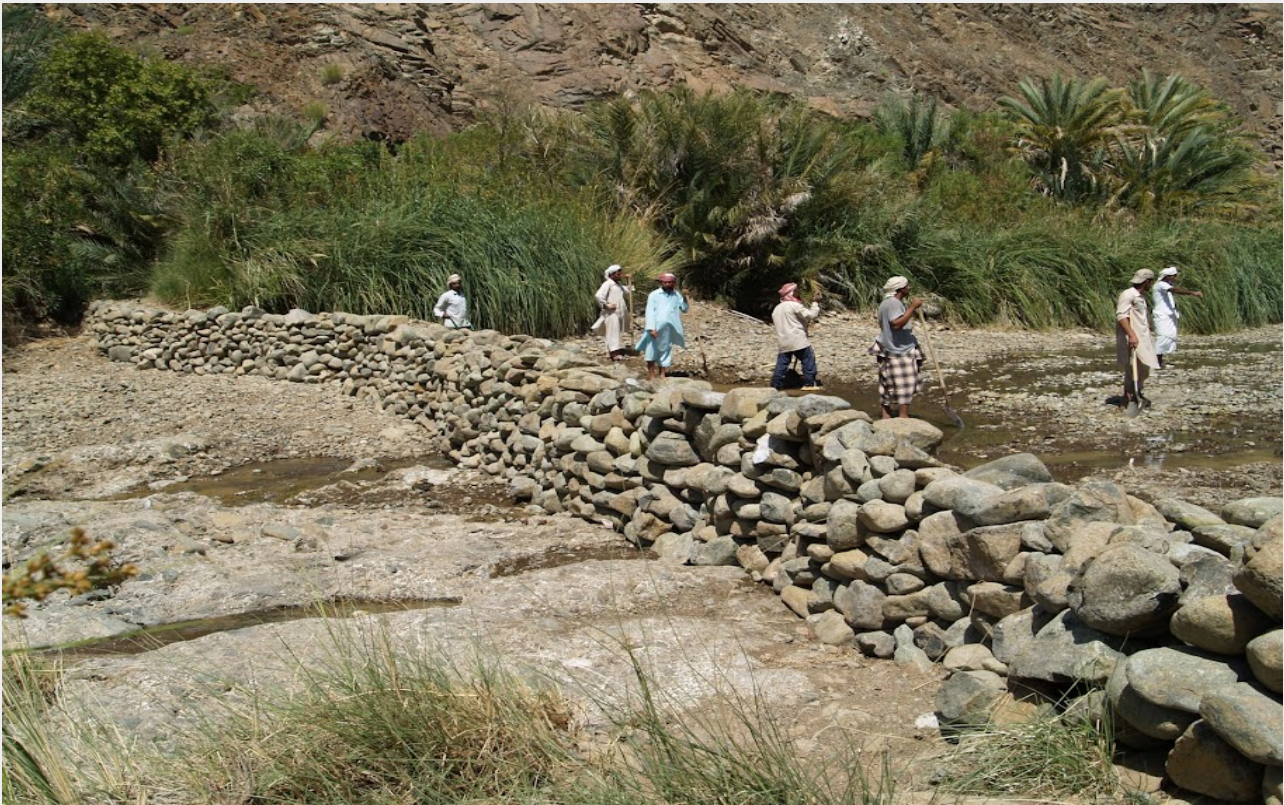
Workers shore up the dam at Wadi Jazira - following a flash flood, the dam was washed away. The photo shows the new dam almost finished; soon a large pool of water will form in the catchment area, which goes to irrigate nearby oases. Please make sure that if there is any sign of rain you do not enter the canyon: seriously.
