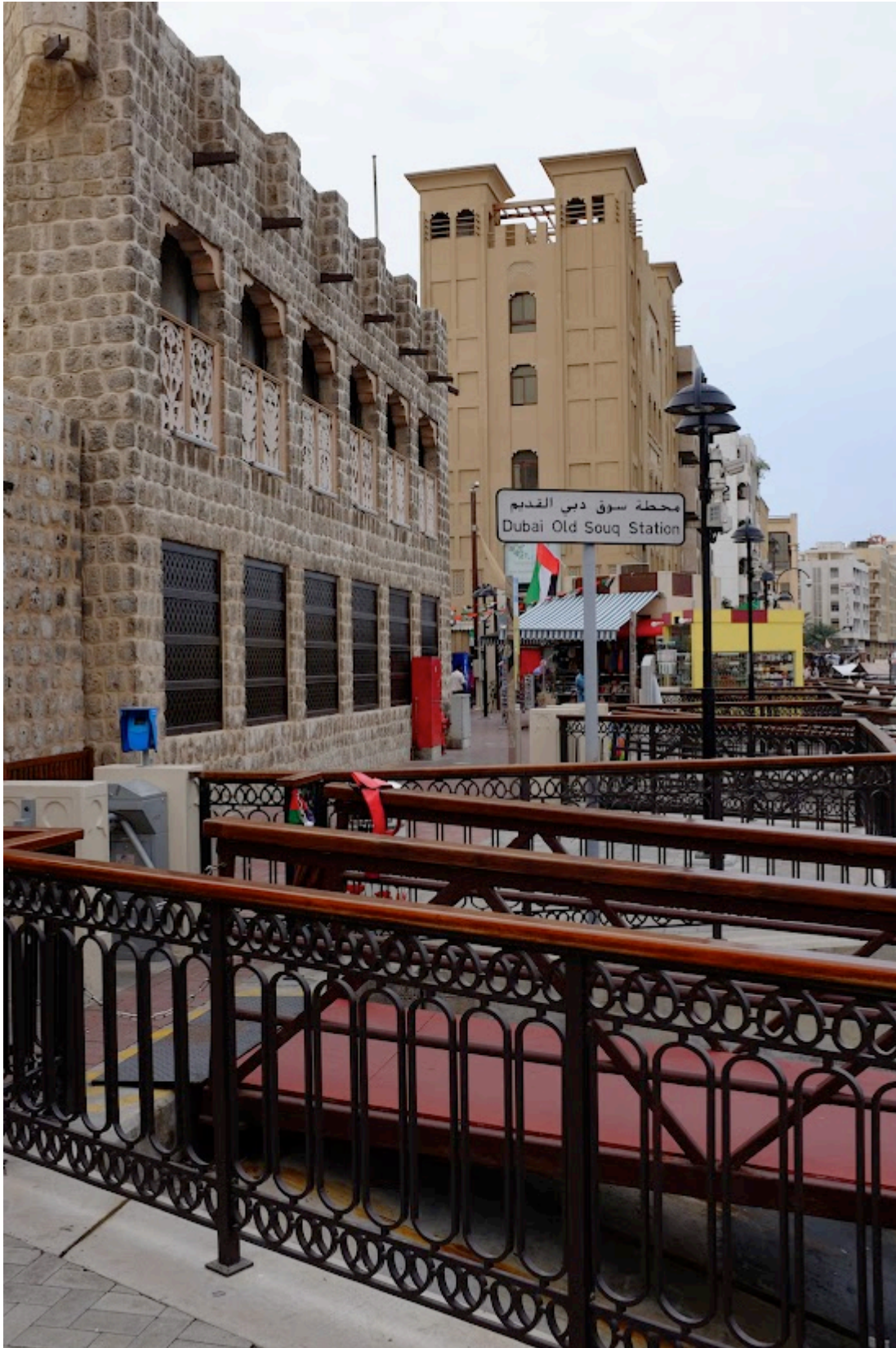
Here the buildings are built with bricks made of sea coral, as they were made traditionally.
